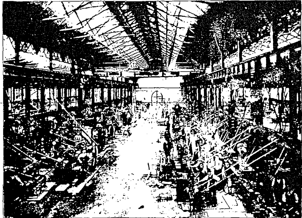
The Turning and Machine Shop.
