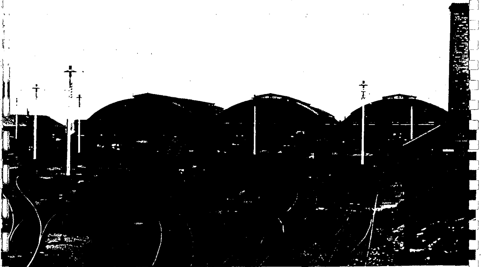
Fig. 10. Railway Running Sheds, Eveleigh 1890's. The building housing the electric light plant with its twin boiler chimneys was erected on the south side of the Running Shed to provide light for overnight servicing of locomotives. The small brick building in the right foreground housed the sand-drying furnace - dry sand is still used on locomotives to assist traction in slippery or icy conditions. (B26)
