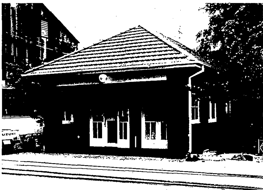
Fig. 52 Carriage Workshops - Ambulance Room Constructed in 1937, this Ambulance Room has thick brick walls, a tiled roof and overhanging eaves to provide a cool and quiet environment for injured or ill workers.
