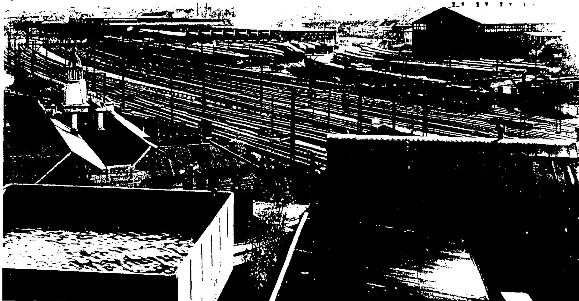
Fig. 50. Carriage Workshops. The extension to the Paint Shop, erected in 1912, was built in corrugated-iron, having a similar design and arrangement as the original, except that the saw-tooth roof was orientated at 90° to the original. The Trimming Department was moved into the enormous corrugated-iron shed at some stage during the 1930's, a temporary arrangement that lasted for the next fifty years. (B 2-9)
