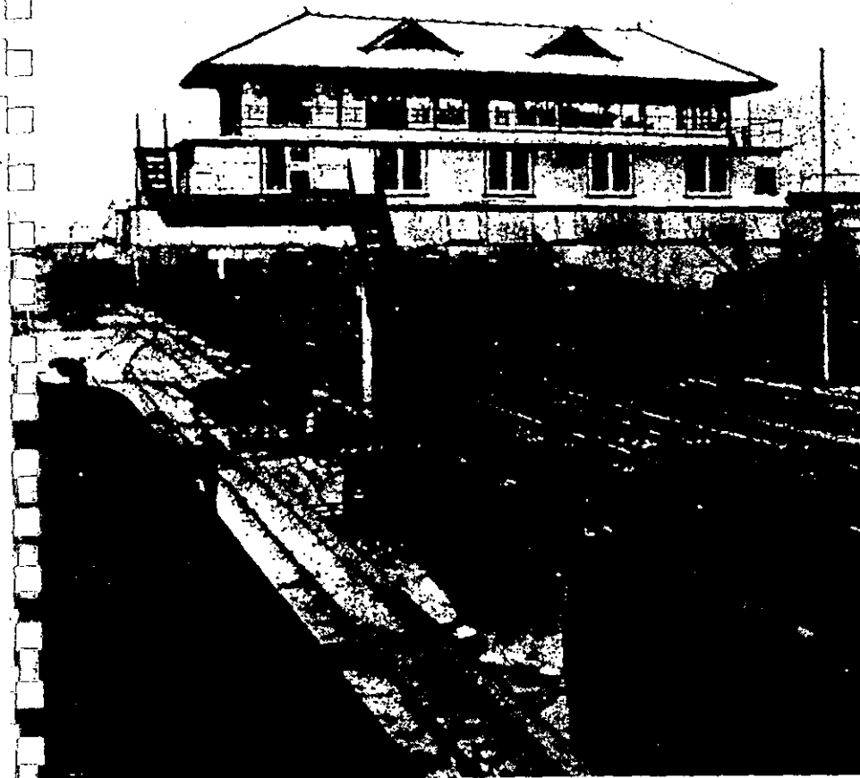
Fig. 45. Eveleigh Railway Yard, Illawarra Junction Signal Box. Following the quadruplication of the main suburban rail lines and the completion of the construction of the Illawarra lines, the Eveleigh Railway Yard became a complicated array of tracks, sidings and junctions leading to the Central Station terminal. The management and safe-working of the yard was conducted from the elevated Illawarra Junction Signal Box. (A9)
