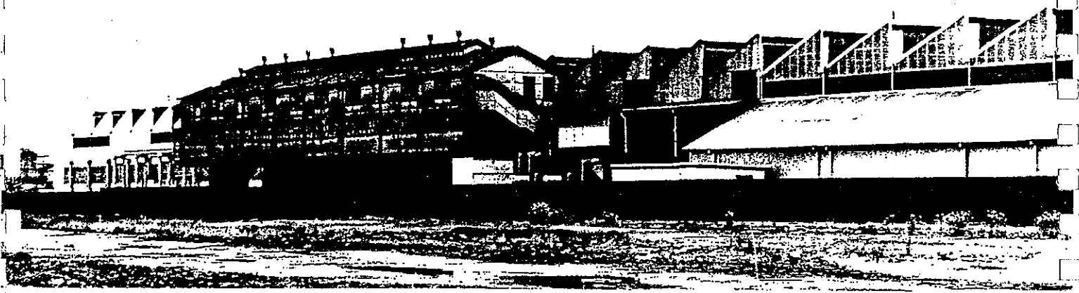
Fig. 57. Loco Workshops, Foundry. In 1944, an extensive staff amenities centre was constructed on the southern side of the Foundry for the foundry staff. Hidden between the foundry and the now demolished Alexandria Goods Shed, little attempt was made to integrate it the existing building design. It was supported on columns above a siding which extended to the Pattern Shop nearby. (W 31)
